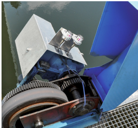
Lubricating bearings via tubes in a secondary clarifier.
